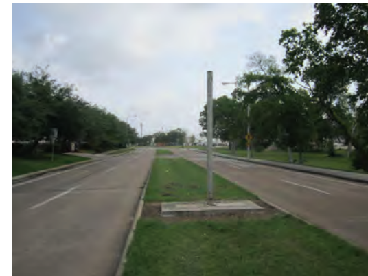
Remaining footing and internal support 7.12
