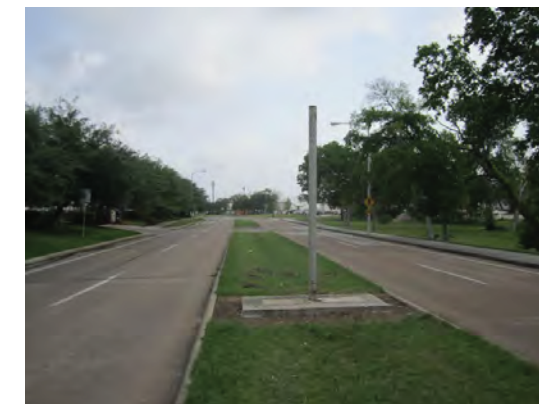
Remaining footing and internal support 7.12
