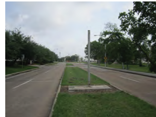
Remaining footing and internal support 7.12
