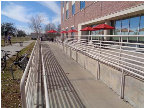
121034a 2/10/2022 ADA-compliant wheelchair ramp and rails Main entrance
