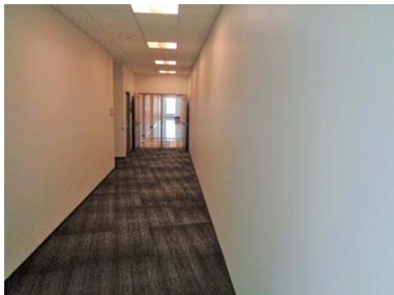
121015a 2/10/2022 Painted hard surface walls Third floor corridor
