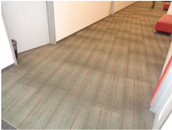
121004a 2/10/2022 Carpet tiles First floor corridor
