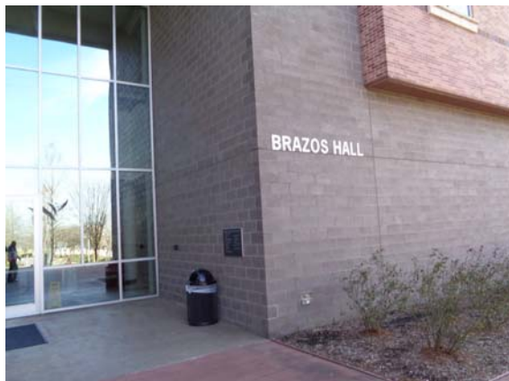
121030a 2/10/2022 Cement masonry block exterior wall North elevation
