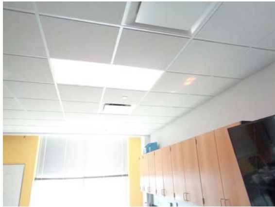
121013a 2/10/2022 Suspended acoustical ceiling Lab 387
