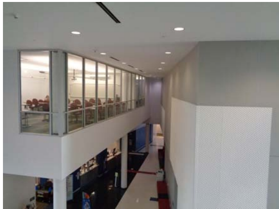
121014a 2/10/2022 Painted hard surface ceiling Second floor, lobby
