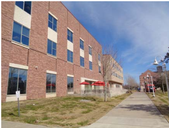
121032a 2/10/2022 Exterior brick wall South elevation
