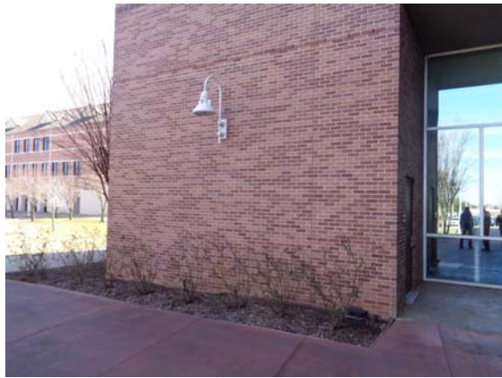
121029a 2/10/2022 Standard brick exterior wall North elevation
