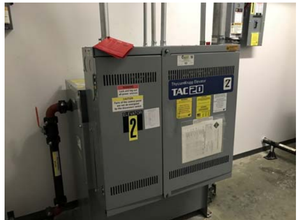
121042e 2/10/2022 Elevator 3 hydraulic controls Elevator mechanical room 158
