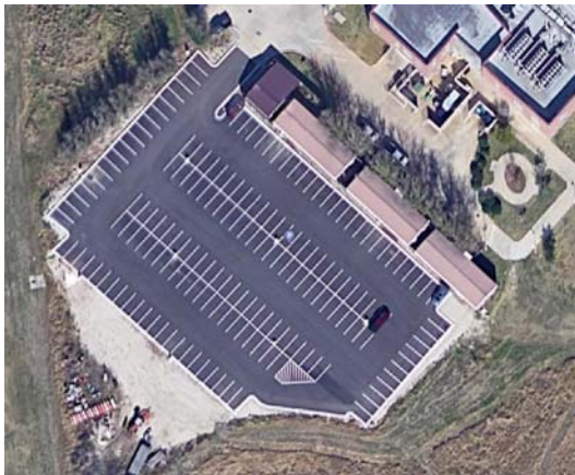
121048a 2/10/2022 Asphalt parking lot Aerial view
