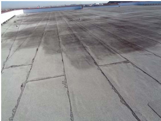
121002a 2/10/2022 Modified bitumen roofing Main roof
