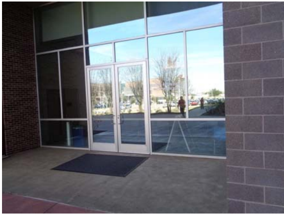
121031a 2/10/2022 Aluminum and glass doors and storefront West elevation
