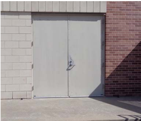
121026a 2/10/2022 Hollow-metal exterior doors Receiving area
