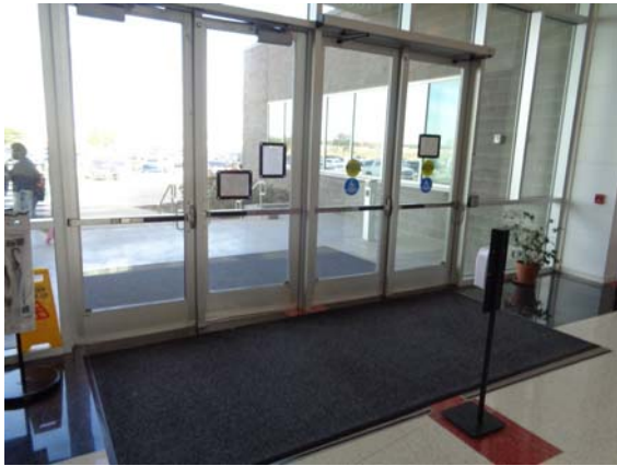
121025a 2/10/2022 Aluminum and glass exterior doors Main entrance
