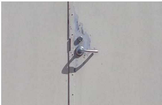
121027a 2/10/2022 Exterior commercial hardware Receiving area
