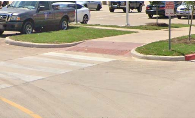
121047a 2/10/2022 Concrete curb and gutter North lot
