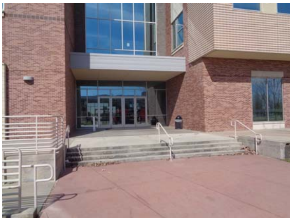
121033a 2/10/2022 Entrance steps and rails Main entrance area
