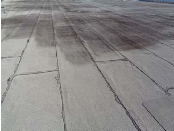
121001a 2/10/2022 Modified bitumen roofing Main roof
