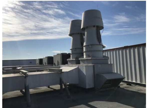
121001e 2/10/2022 Mixed flow, short stack exhaust fans Roof
