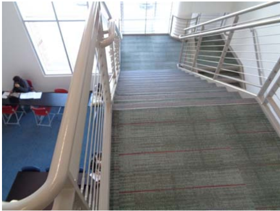
121010a 2/10/2022 Carpet stair treads Stair A1
