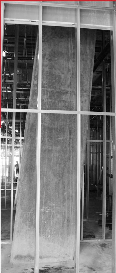
Even the support structure for the new building required a specialized design. The foundation for Armistead prevented the support columns for HBSB II from being vertical, so they were instead installed at an angle. The columns are just as sturdy and will be unnoticeable when the building is complete.
