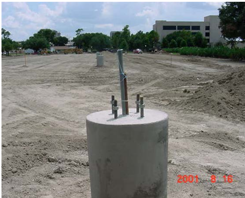
FIGURE 9.9.5 CONCRETE LIGHT POLE BASE WITH ANCHOR BOLTS
