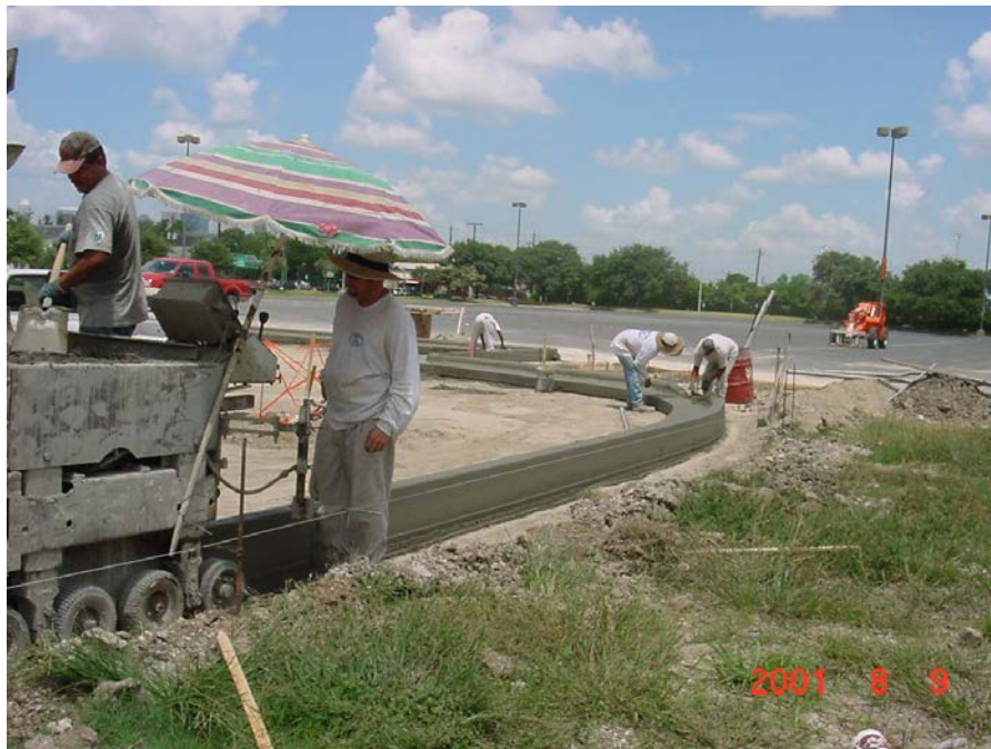
FIGURE 9.2.8 MONOLITHIC CURB ALONG PERIMETER OF PARKING LOT
