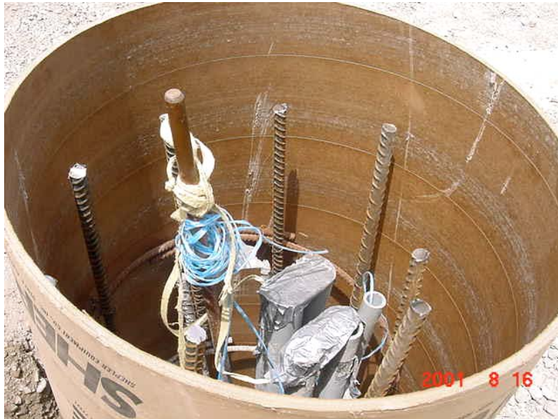
FIGURE 9.9.4 REBAR, ELECTRICAL CONDUIT
