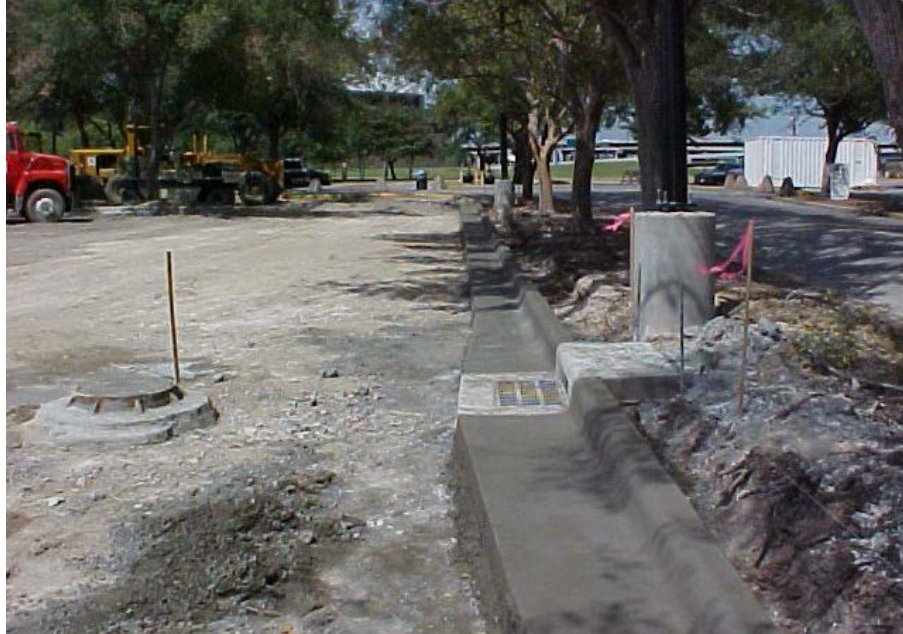
FIGURE 9.8.2 MONOLITHIC CURB, INLET AND CATCH BASIN
