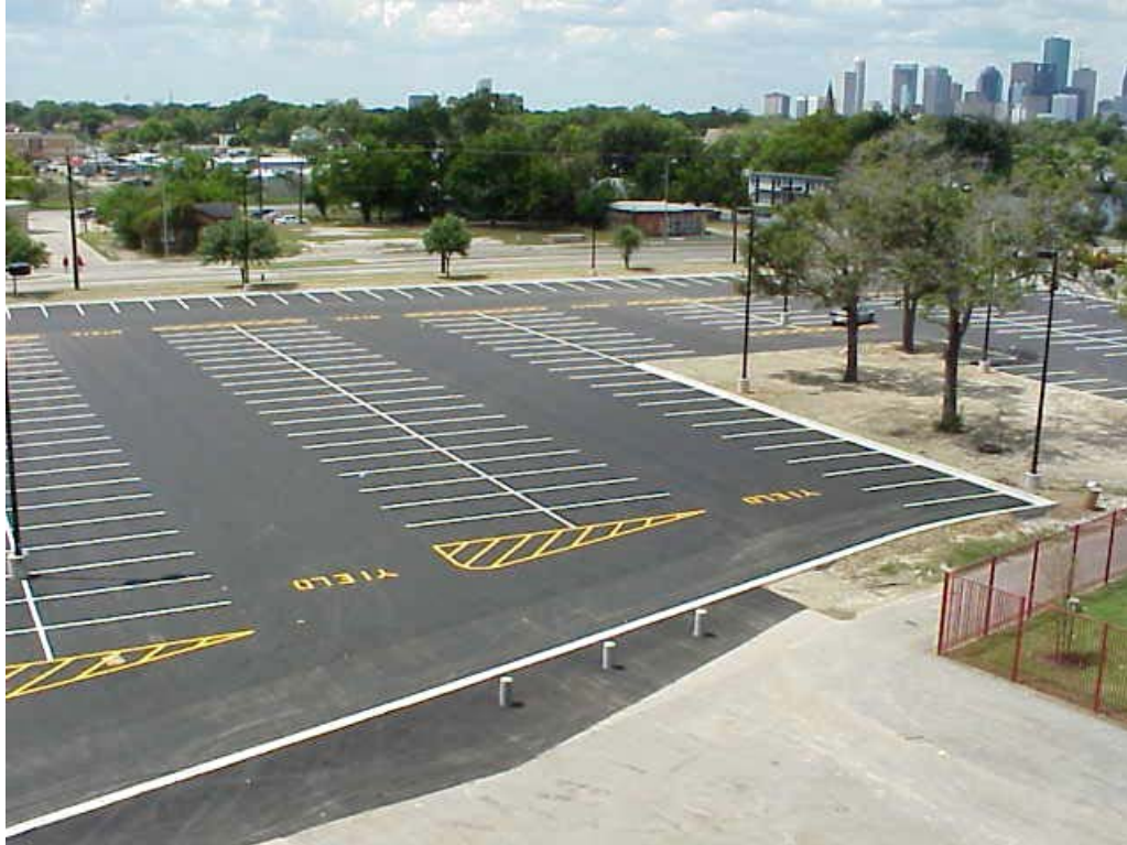
FIGURE 9.2.5 PERPENDICULAR (90°) PARKING SPACES
