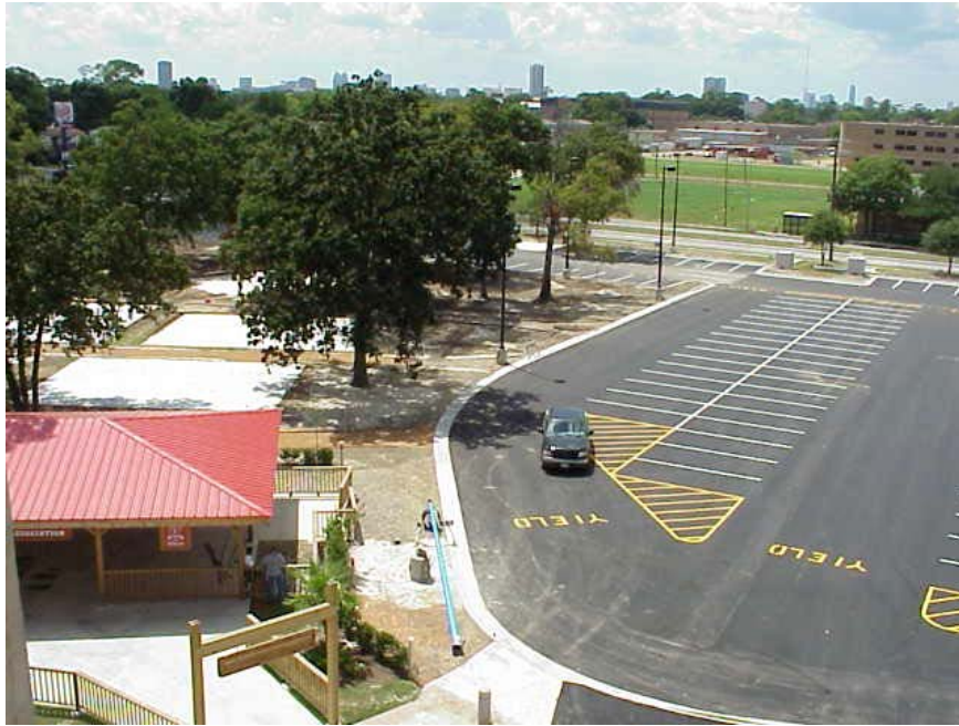
FIGURE 9.10.2 YIELD MARKINGS AND YELLOW STRIPING
