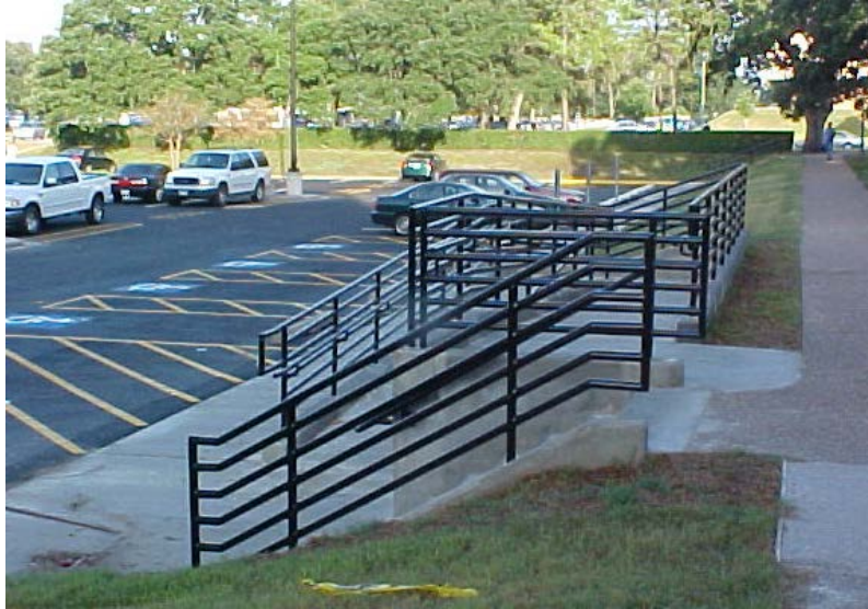
FIGURE 9.3.1 SHARED HANDICAPPED ACCESS AISLES LEADING TO RAMP
