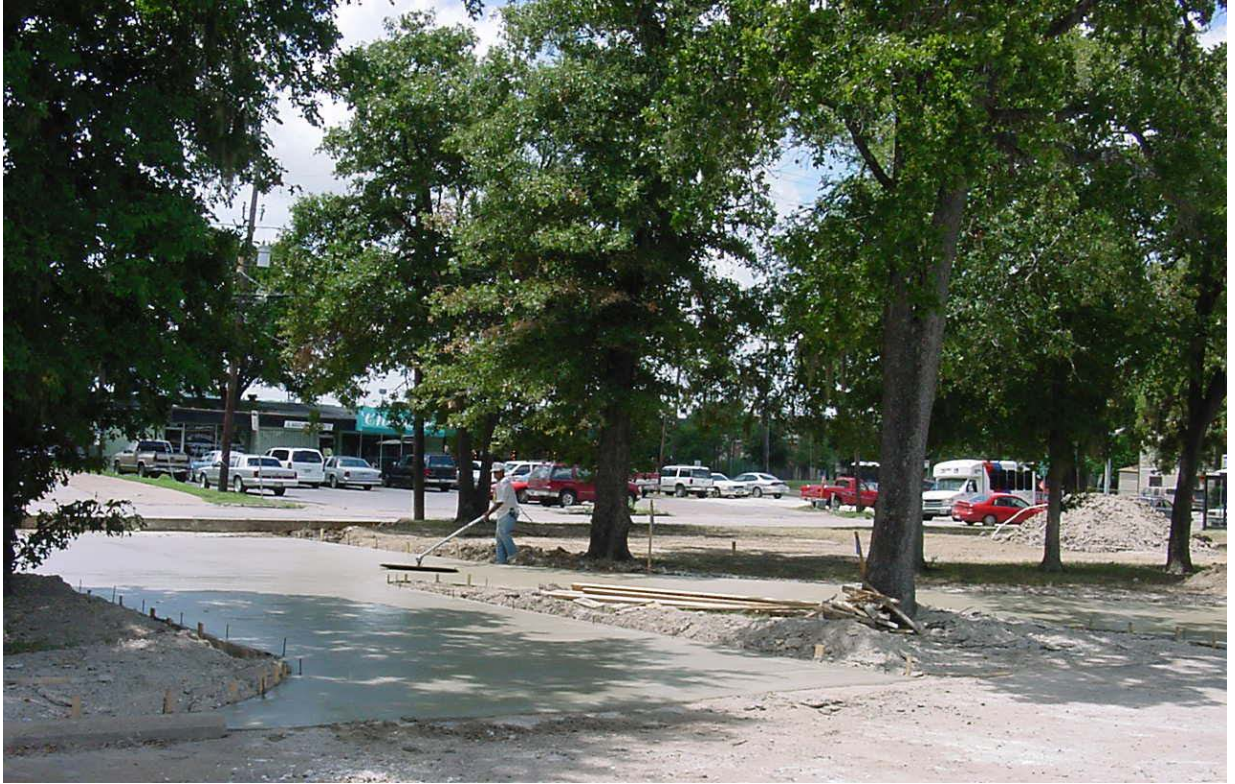
FIGURE 9.2.2 FINISHING CONCRETE AT WHEELER STREET DRIVEWAY
