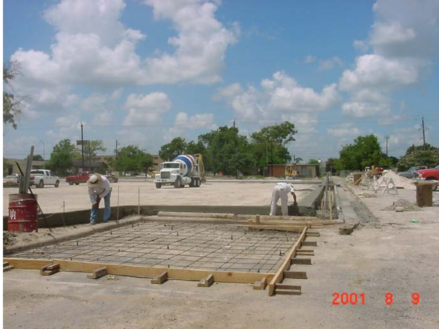
FIGURE 9.6.1 FRAMING AND REINFORCING FOR CONCRETE PAD
