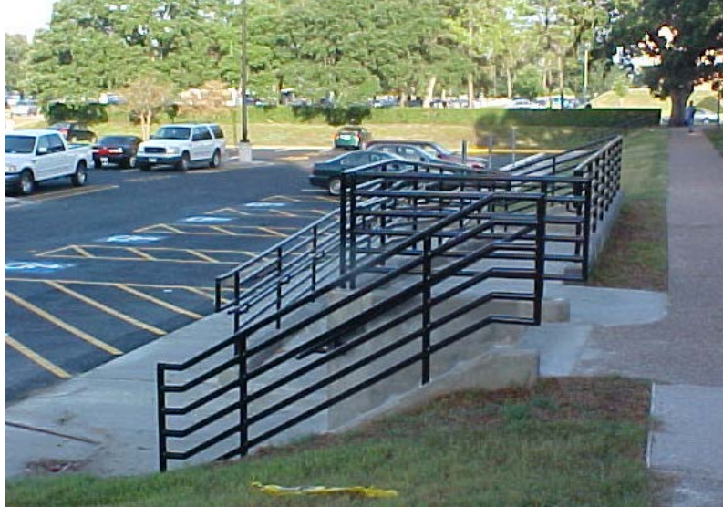
FIGURE 9.3.1 SHARED HANDICAPPED ACCESS AISLES LEADING TO RAMP
