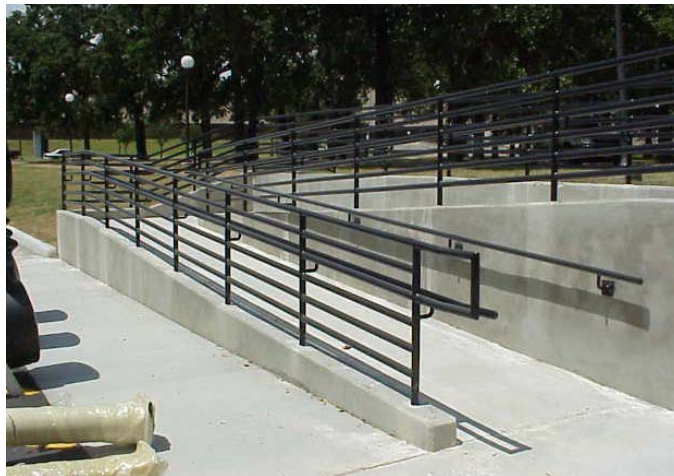
FIGURE 9.3.4 ADA RAMP AND HANDRAILS
