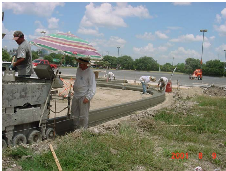
FIGURE 9.2.8 MONOLITHIC CURB ALONG PERIMETER OF PARKING LOT
