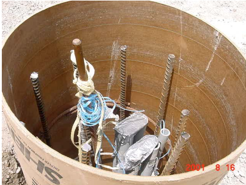
FIGURE 9.9.4 REBAR, ELECTRICAL CONDUIT
