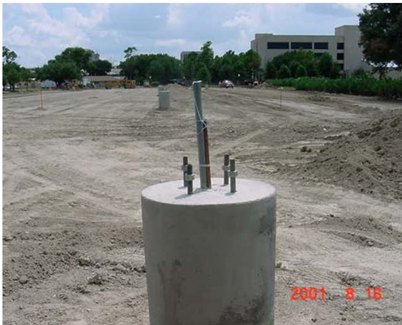
FIGURE 9.9.5 CONCRETE LIGHT POLE BASE WITH ANCHOR BOLTS
