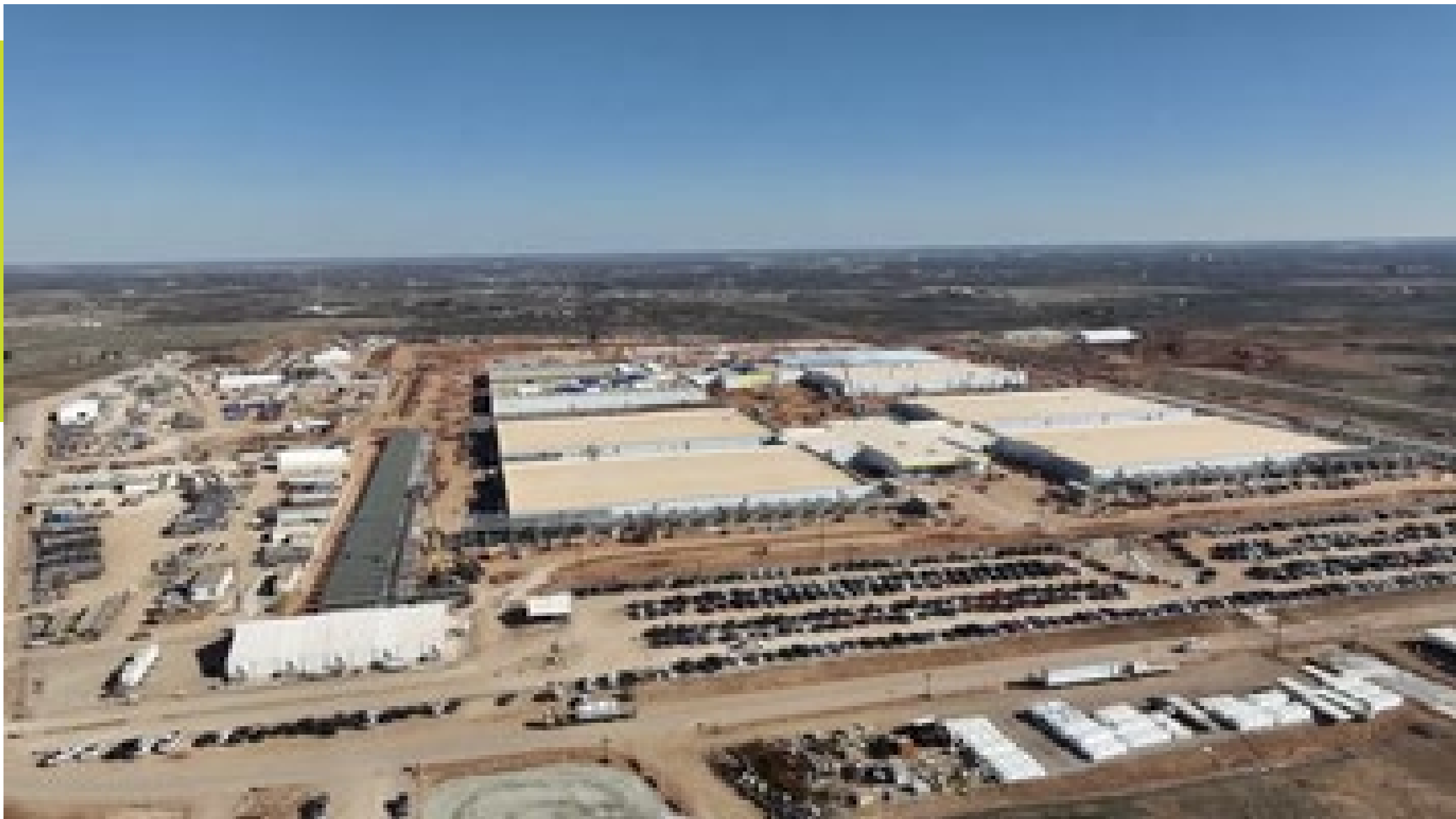
OpenAI Stargate facility in Abilene, TX (Data Center Dynamics)
