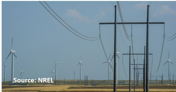
Electrification – One Key to Decarbonization
