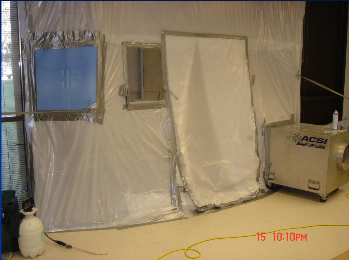
Large (> 25 square feet) Abatement Procedure in Progress
