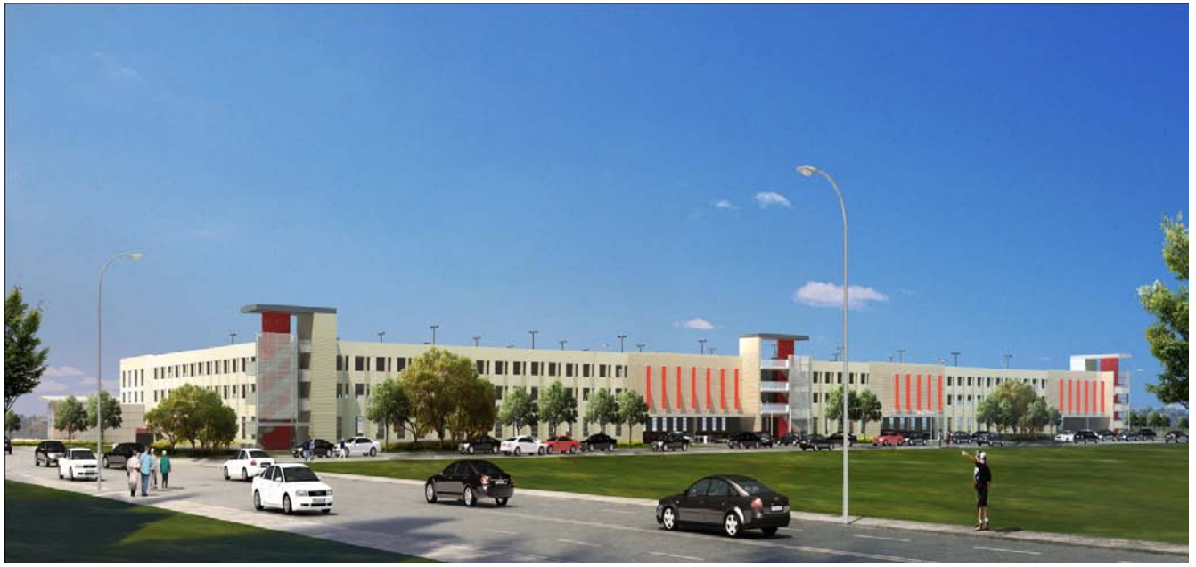
Stadium Parking Garage – Northeast View from Cullen and Holman
