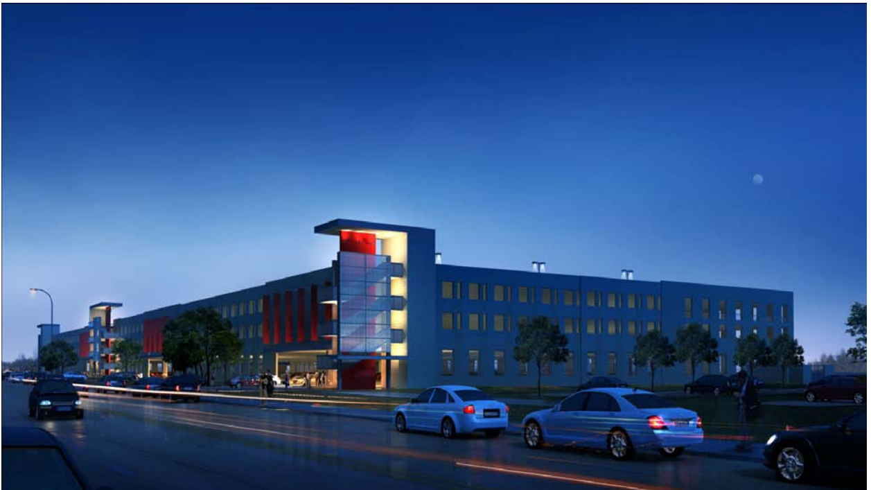
Stadium Parking Garage – Along Holman Street
