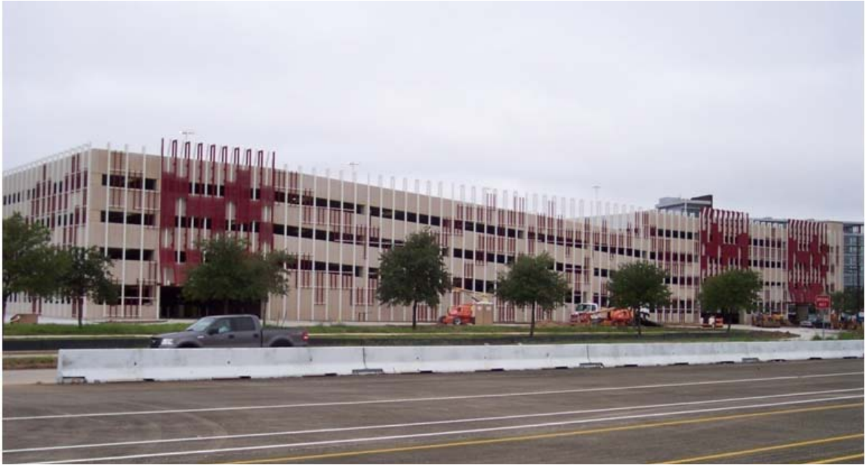
East Parking Garage – Eastside along Spur 5
