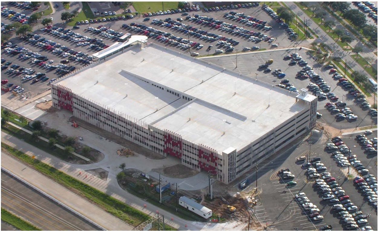
East Parking Garage – Aerial View
