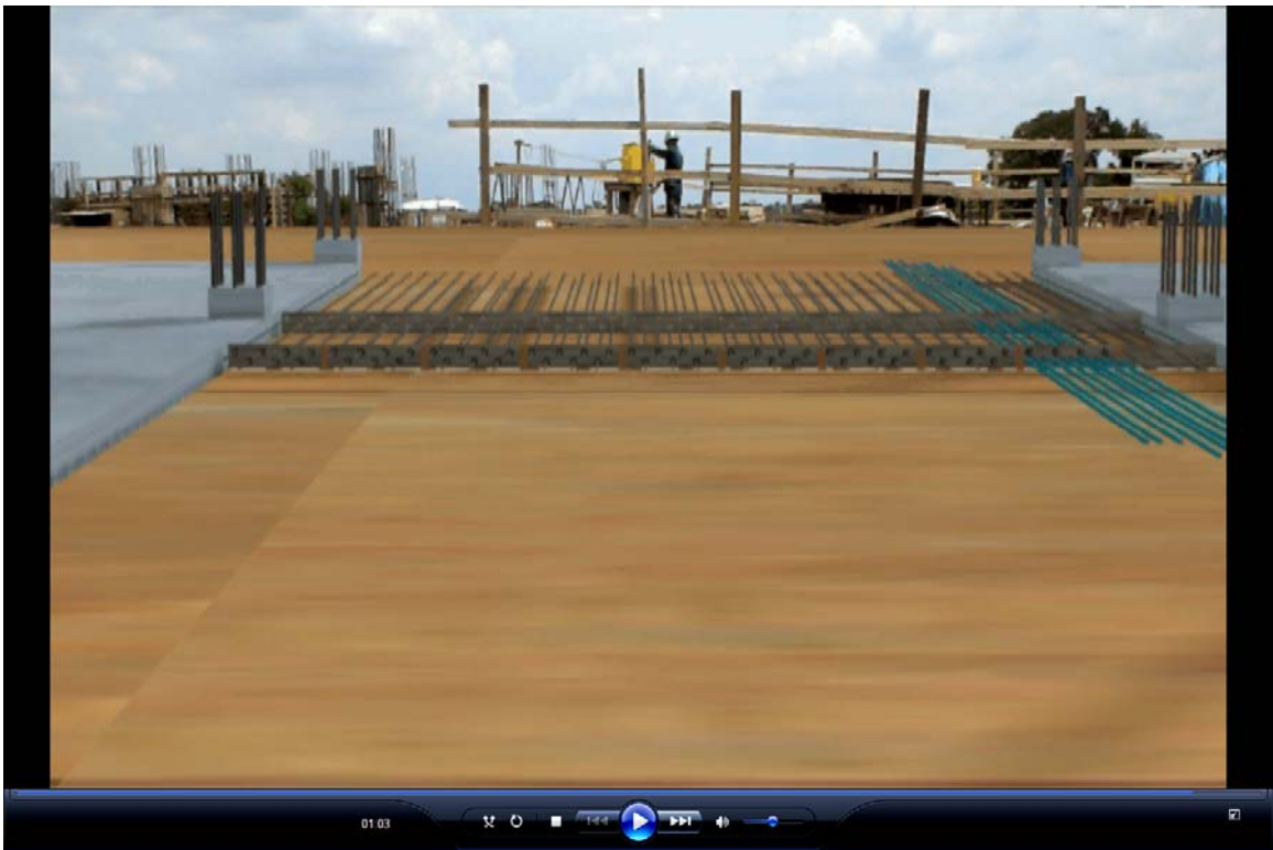
Figure 17: The final completed installation
