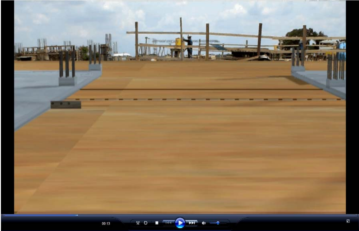
Figure 14: Bulkhead being marked for drilling holes for rebar
