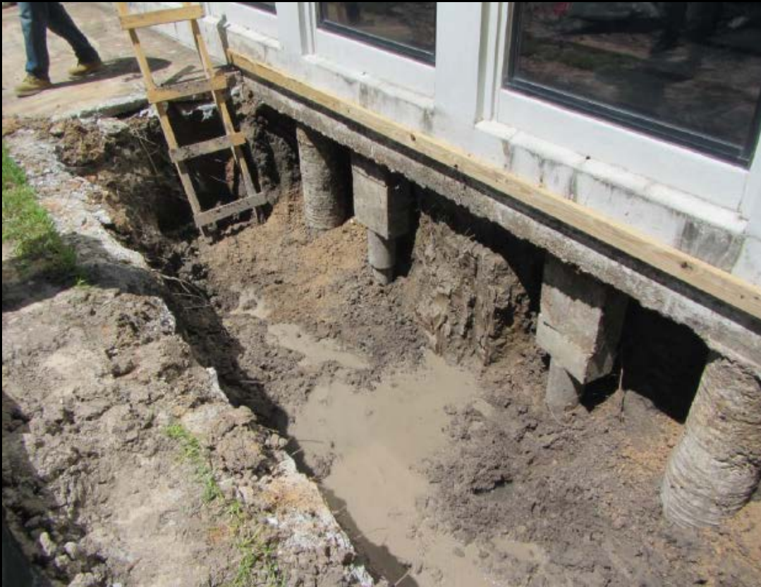
Seepage from under the building saturated soil
