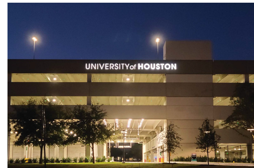
CAMPUS PERIMETER ILLUMINATED IDENTIFICATION AS INSTALLED AT THE ELGIN STREET GARAGE. Example shown does not reflect correct typography
