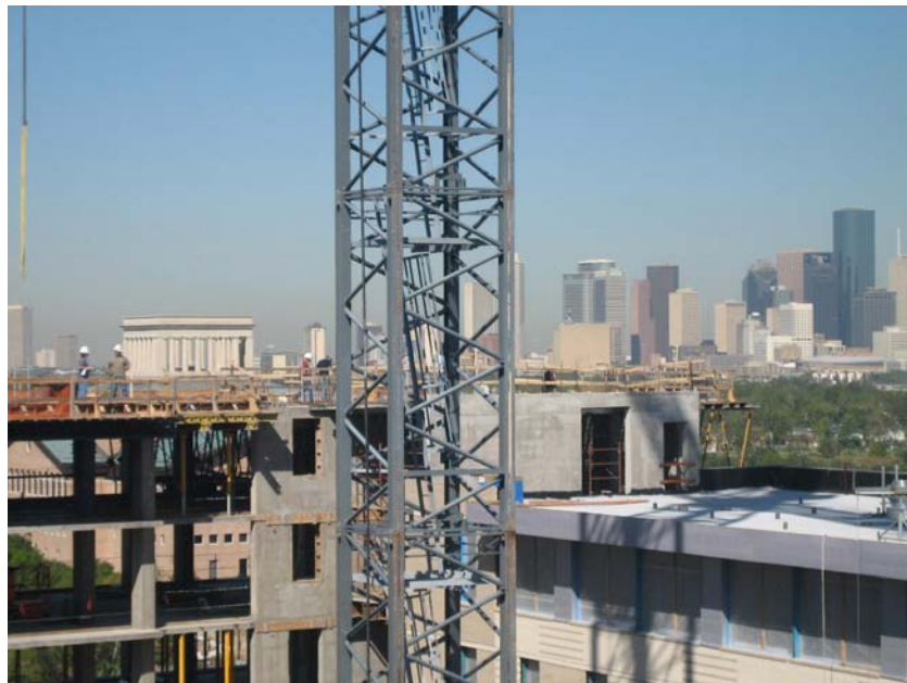
Calhoun Lofts construction site buzzes with activity
