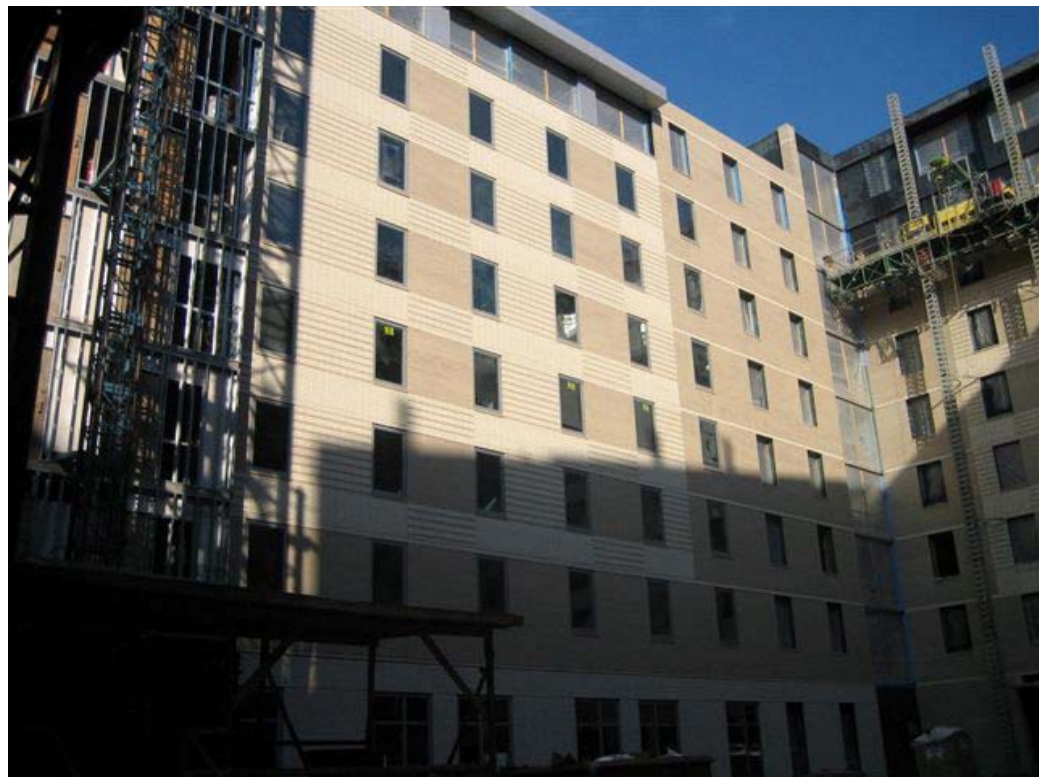
South face of North Building Completed Masonry
