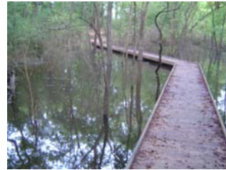
Figure 2- Boardwalk crossing over Wetlands
