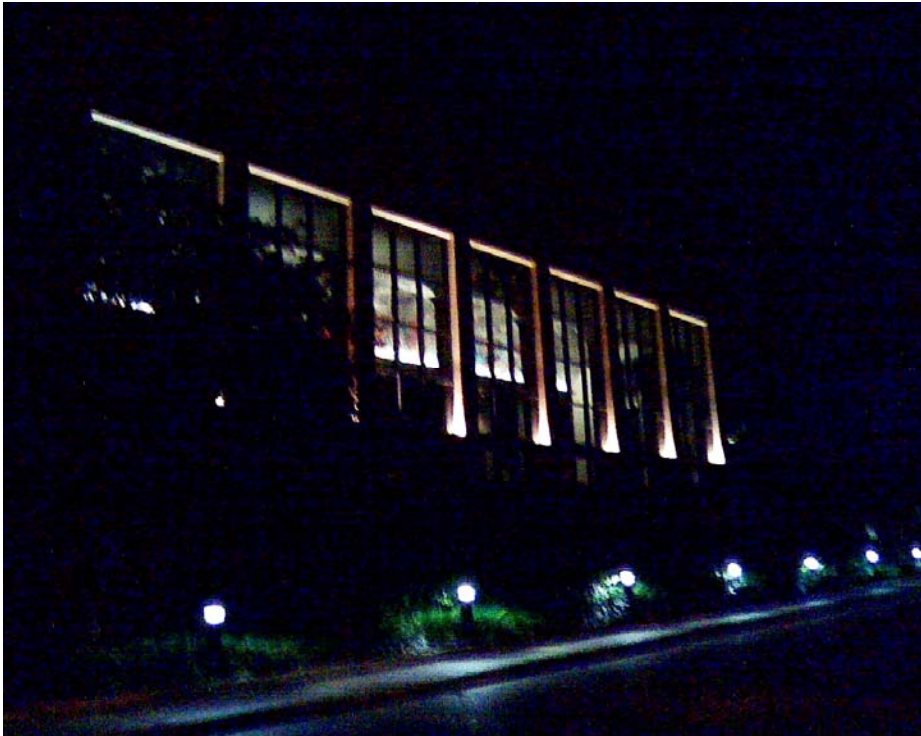
Lighting improvements near Moores School of Music
