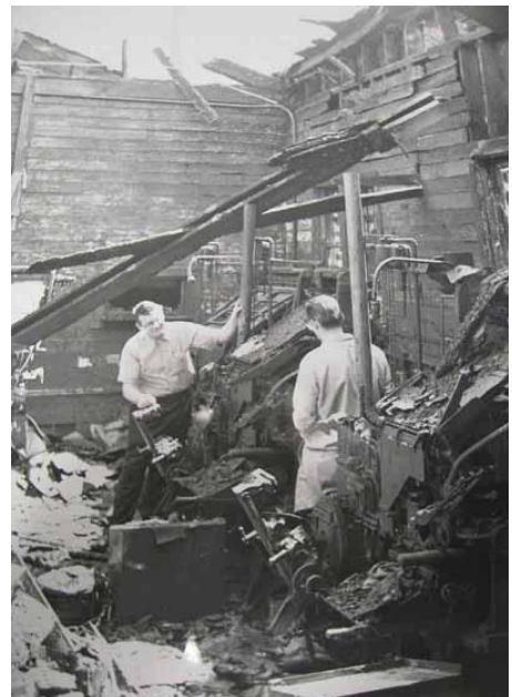
Damage after 1960 Fire
