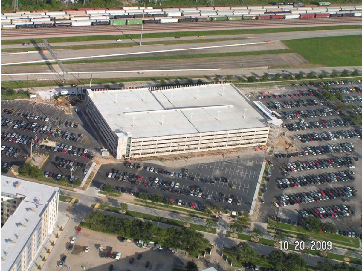
Aerial View of East Parking Garage taken October 20, 2009
